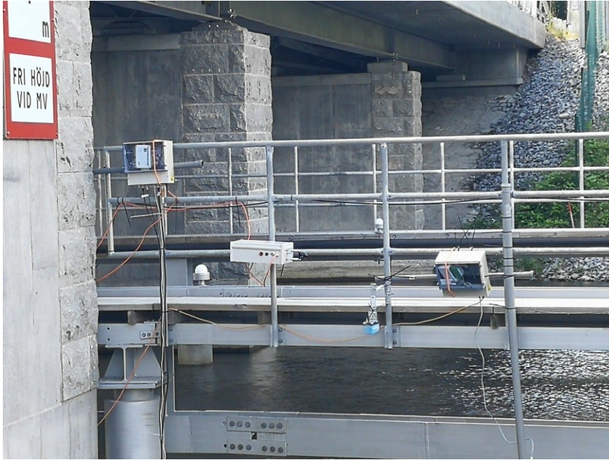
Figure 15: All water sensors installed at the Flottsund bridge in Uppsala. Image courtesy of RISE AB. From left to right: 1. 3G sensor box / water hydrostatic level (depth) / pH / TDS-Conductivity / water temp / air temp-humidity (RISE). 2. Turbinator (IVL) 3. Water level radar (RISE) 4. Conductivity (Talkpool). Image courtesy of Dimitar Kolev, RISE AB
